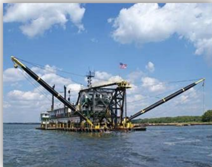
Brunswick Channel Dredging
