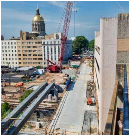
Courtland Street Bridge Replacement - Atlanta
