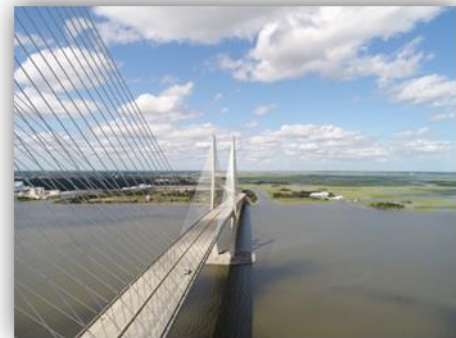
Drone Inspecting Sidney Lanier Bridge after Hurricane Irma
